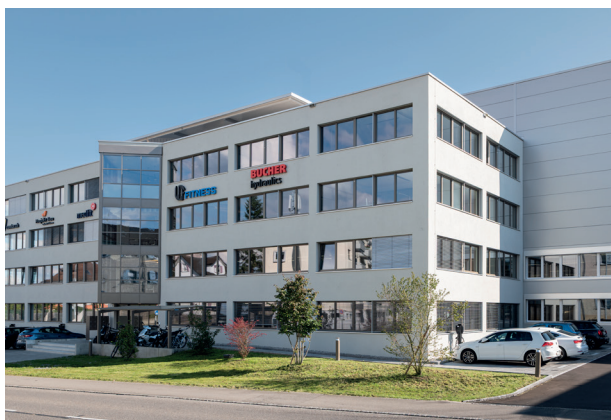
Standort Mobile Drives in Romanshorn.
